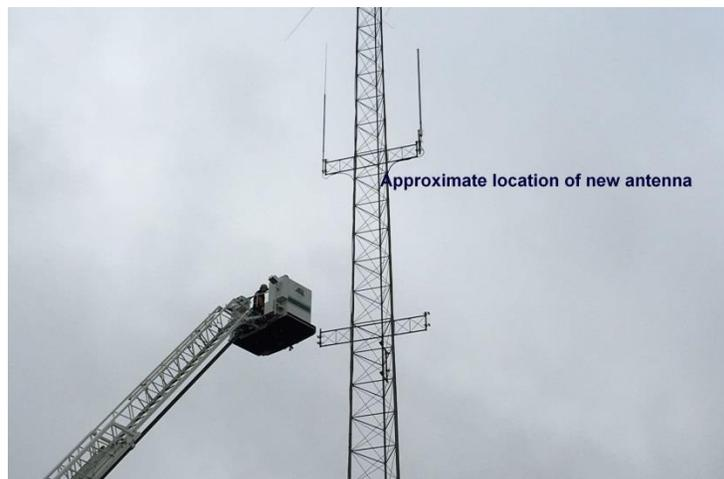
The new D-Star antenna would have its base at about 90 feet above ground level with the antenna tip at about 110 feet above ground level. It would be mounted on the south tower leg off an extension arm.
